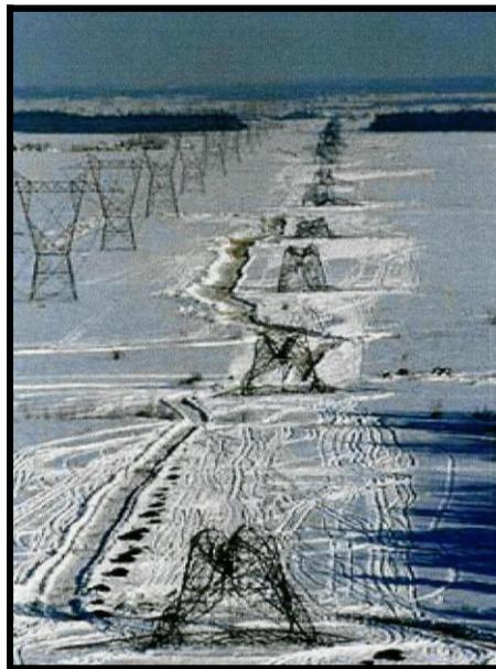
Figure 2.4 – A 735 kV Line Cascade
