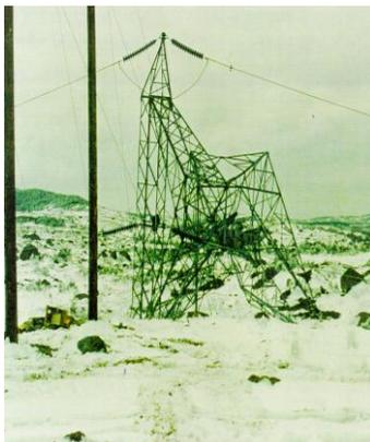
Figure 2.3 – Large Angle Tower Failure near Hawke Hill (1988 Storm)
