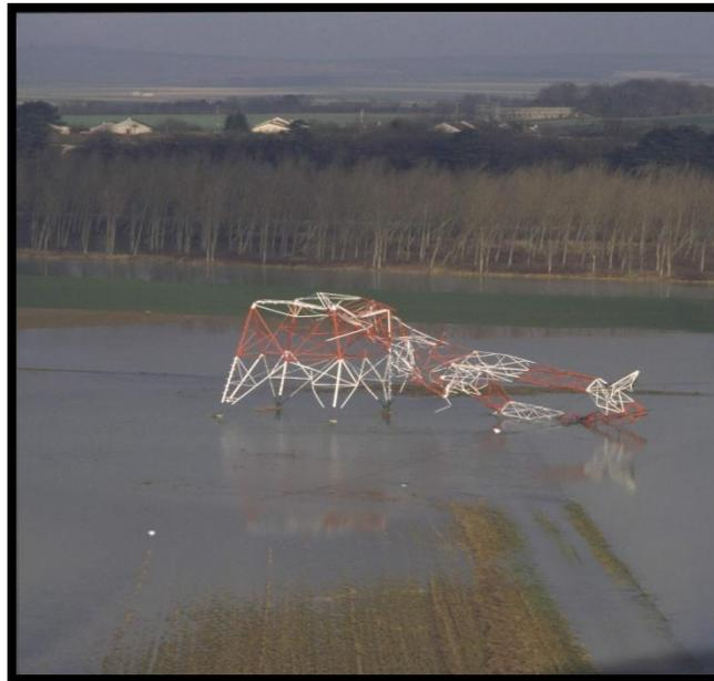
Figure 2.6 – Tower Failure in EDF System (Storm 1999)
